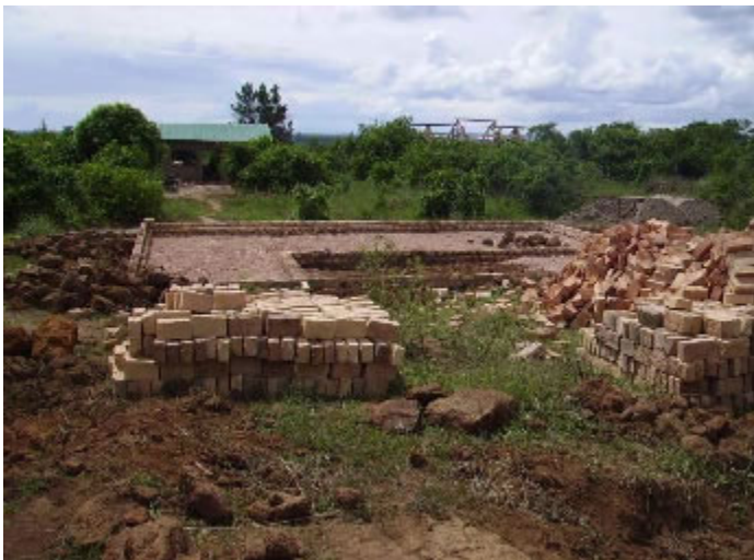
Foundation for the House Parent's house at EWCV, Uganda
