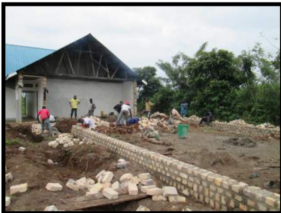
Senior 4 classroom and library foundation Dec. 2 nd .
